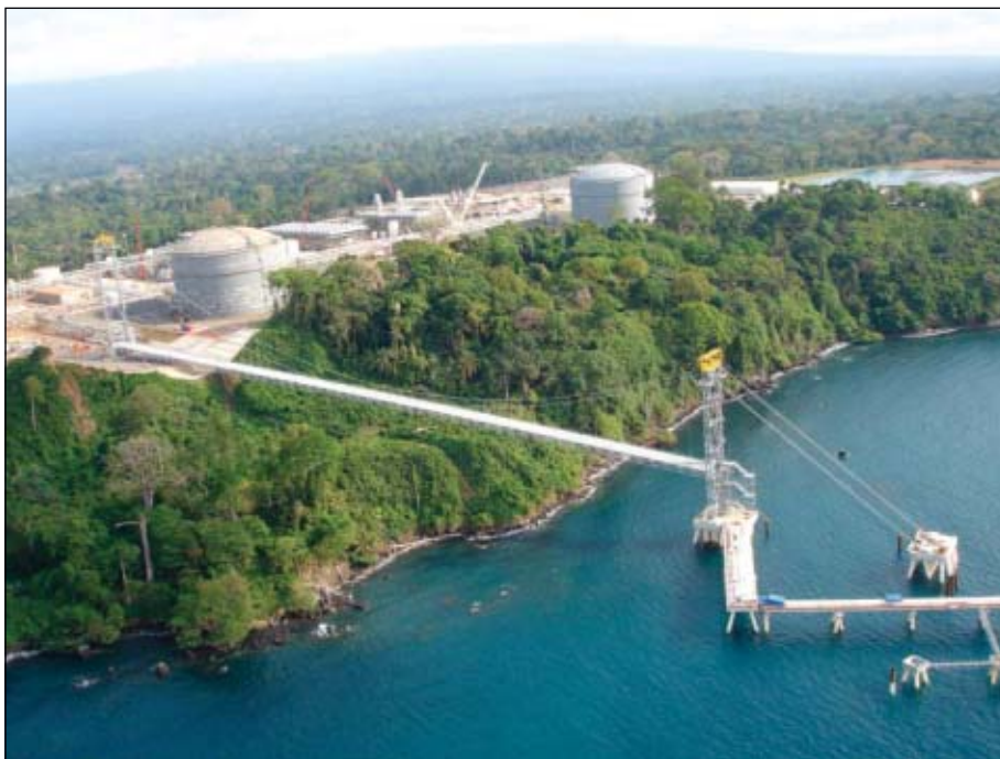
At the end of May, Equatorial Guinea LNG Holdings Ltd. delivered the first cargo of LNG from EG LNG Train 1 on Bioko Island, Equatorial Guinea, into the 138,000-cu m Gracilis under a long-term agreement to supply 3.4 million tpy to BG Gas Marketing Ltd. The cargo was destined for Lake Charles, La. (Photograph from Marathon Oil Corp.)
